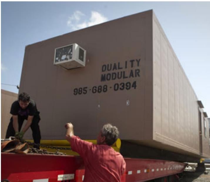
Modular data centers use techniques including preconfiguring a shipping container with server racks and other IT equipment for easy drop-off and deployment. Photo credit: Lee Celano / Reuters
