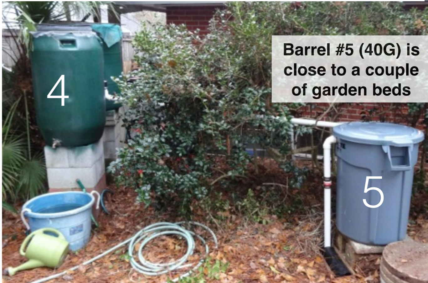
Gravity fill barrels close to garden bed to expand rain water storage capacity and speed up watering
