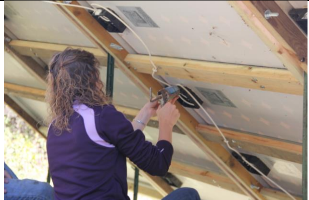
Hannah caulking to keep the water out.
