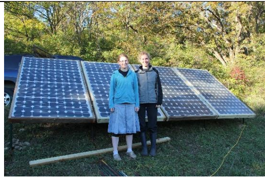
There! The solar panels are all mounted.
