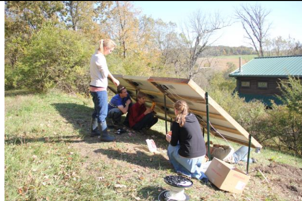
Beginning to wire the panels together with friends to help.
