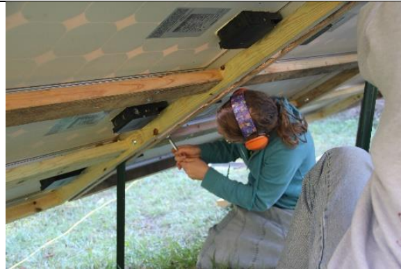
Measuring to mount the unit at the right angle.
