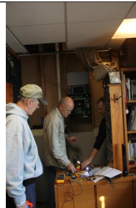
Meanwhile, the electricians are wiring the inverter inside.
