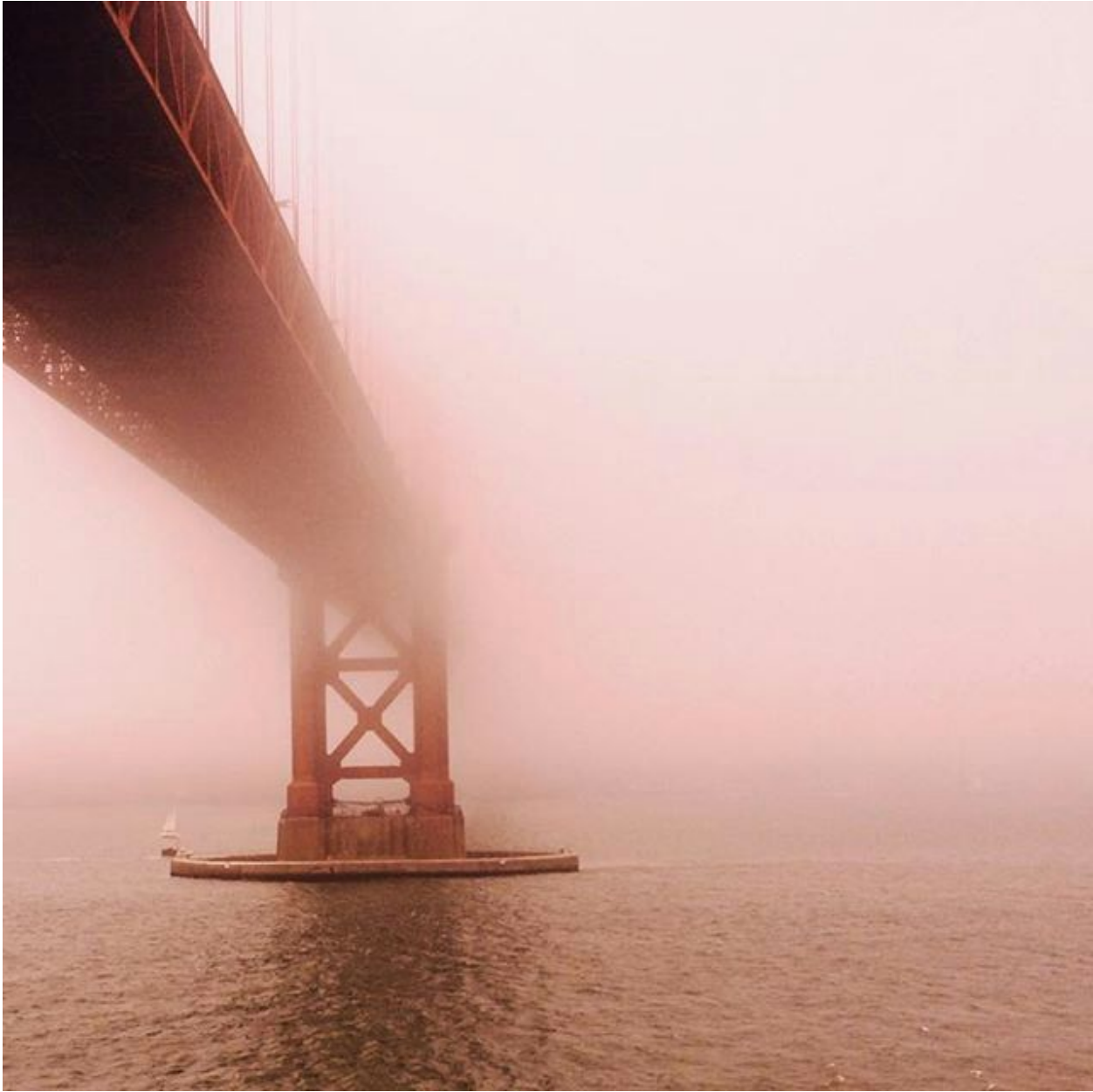
Golden Gate Bridge
