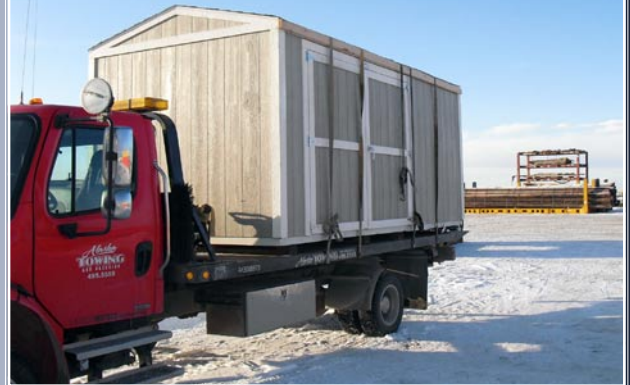
Installed and ready for final grade
