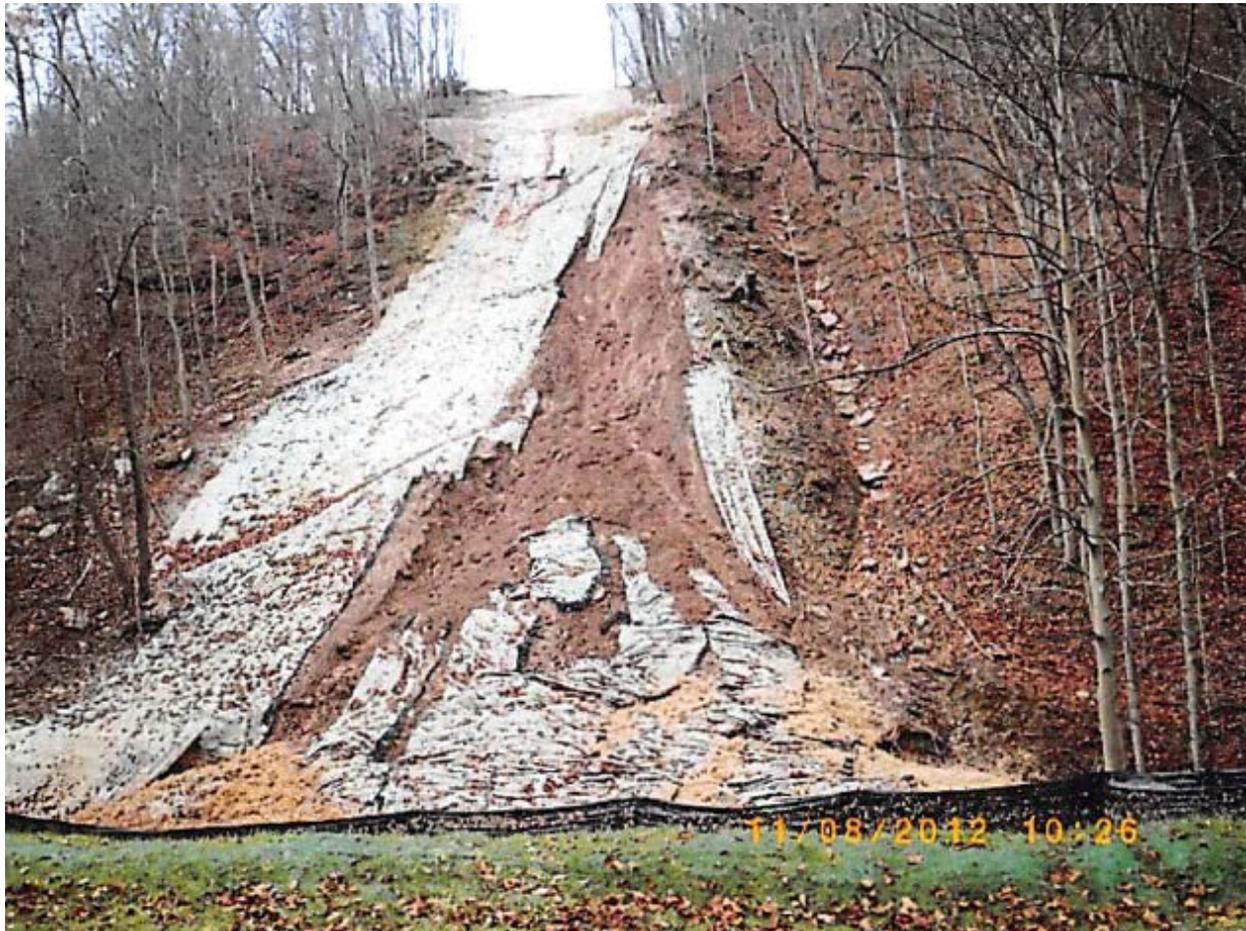
**This photo from West Virginia regulators shows the failure of erosion controls.**
