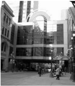
Picture 1 - Two Plus 15 bridges in Calgary. The one in the foreground is an enclosed glass bridge. The bridge in the background is an open bridge with a canopy protecting its users from rain and such but is not heated.
