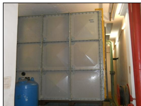
Kirana Residence Domestic Water Retention Tank
