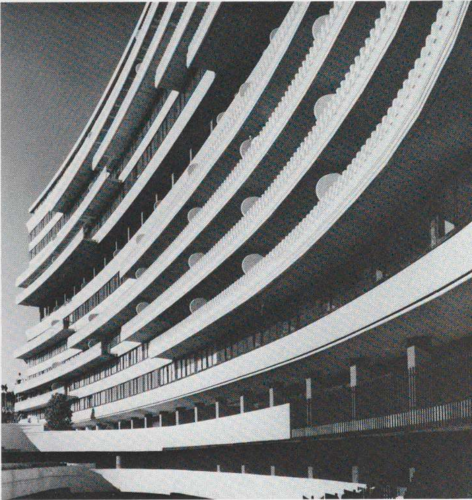
260. Luigi W. Moretti; Fischer-Elmore Associated Architects. The Watergate Apartments, Washington, D.C. 1961-64/70
