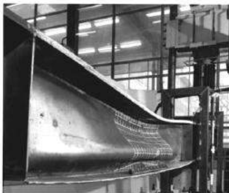
Figure 2. Vertical web buckling.
