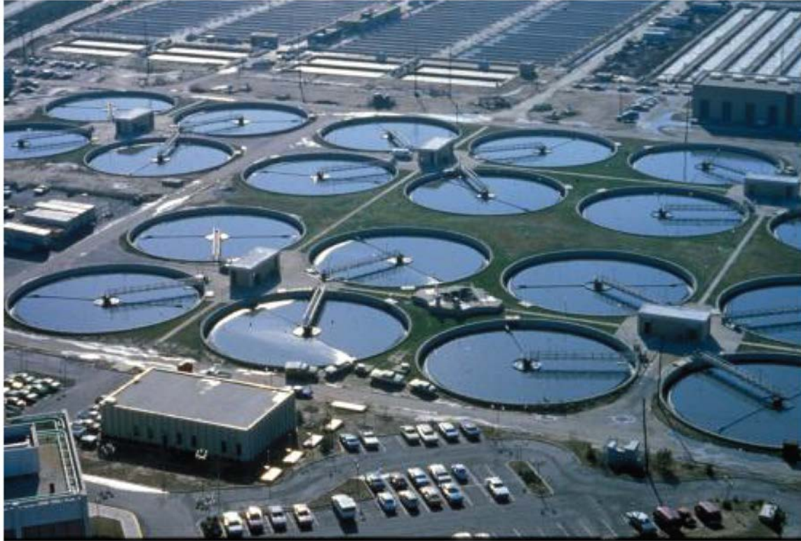
Figure 25.1 Sewage Treatment Plant (credit: "eutrophication&hypoxia"/flickr.com)
