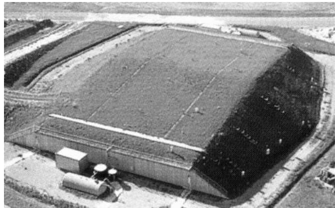
Figure 20b. Experimental cover at Aube disposal facility for medium and low level waste
