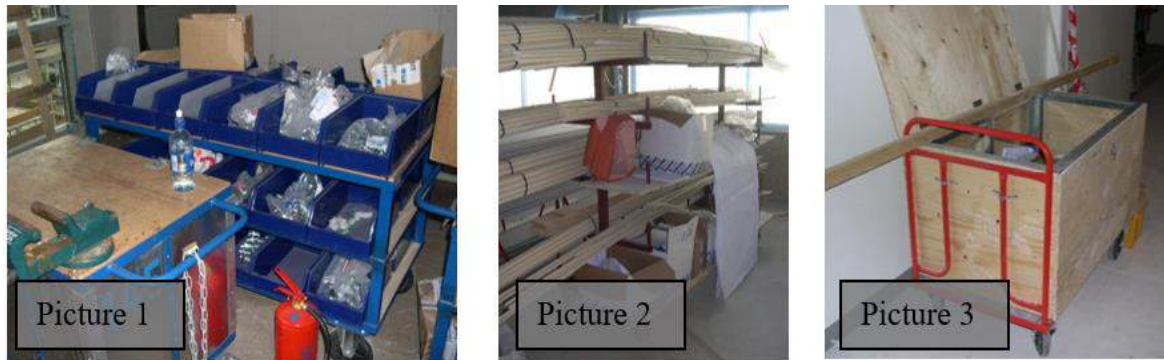
Figure 6 Examples from a project that challenged with the principle "everything on wheels". Picture 1 Both workstation and part storage, picture 2 Larger trolleys used for electrical tubes, metal stud and mouldings. Picture 3. More standard solution. (Photo: J.S)
