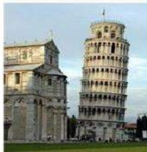
The Leaning Tower of Pisa leans due to a faulty foundation.
