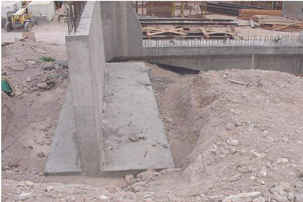
Figure 8-5. Abutment/wingwall footing, I-10, Arizona.
