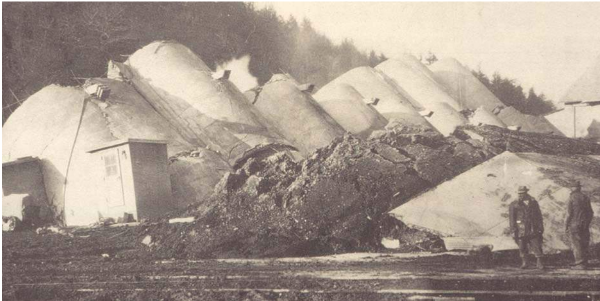
Figure 8-12. Bearing capacity failure of silo foundation (Tschebotarioff, 1951).
