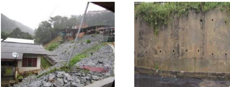
Figure 7. Rubble pitching and retaining wall at Lenggong, Perak
