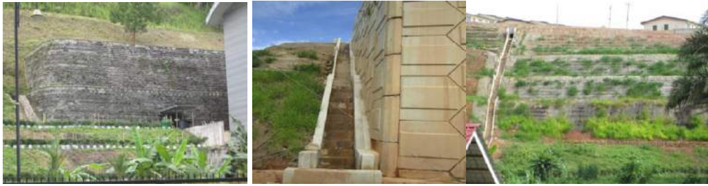
Figure 8. Rubble Pitching, Earth reinforced retaining structure and turfing of slope surface
