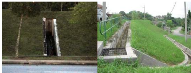
Figure 5. Surface Drainage at Tanjung Malim and Batu Gajah, Perak
