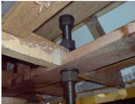
Figure 35-12 Mounting bolt connection
