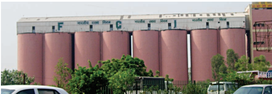
Fig. 1.10 (a) : Silos for storage of grains
