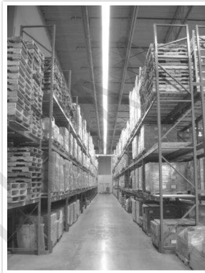
FIGURE 9: Single-Deep Pallet Racks
