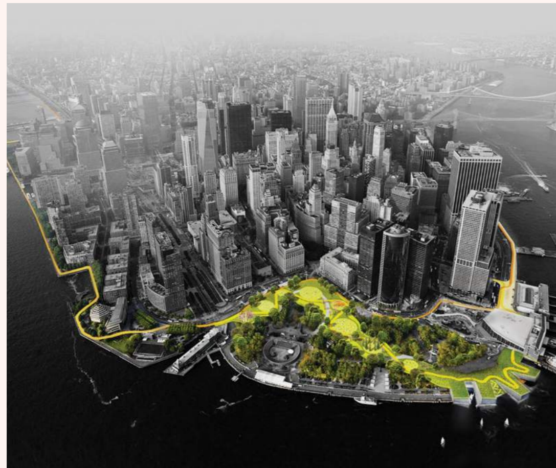
The design of the “BIG U” has fostered community engagements, kept the waterfront safe and is accessible yet inclusive. Source: Rebuild By Design/The BIG Team
