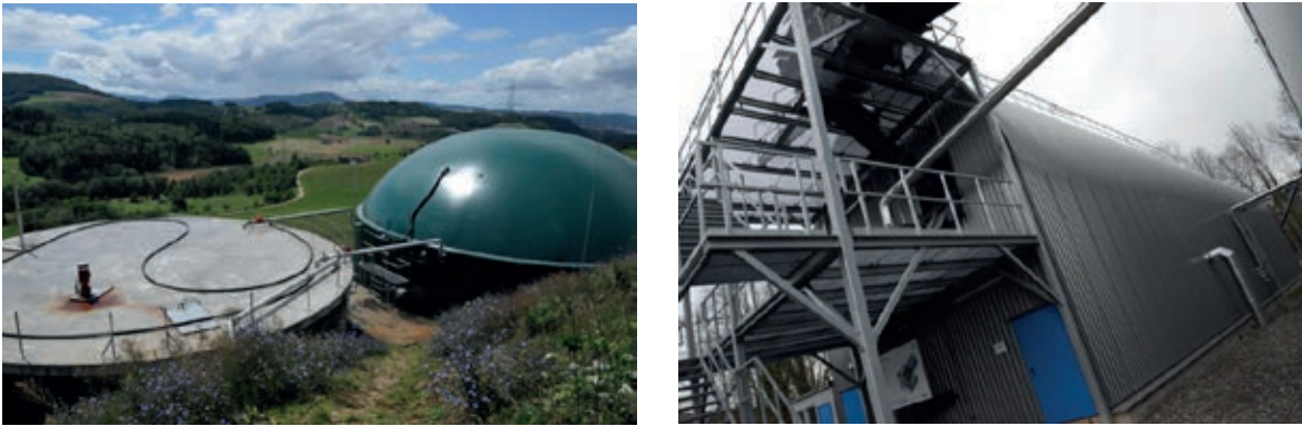
Figure 7.2 View of a mesophilic anaerobic co-digester (left) and an industrial thermophilic anaerobic digester (right).
