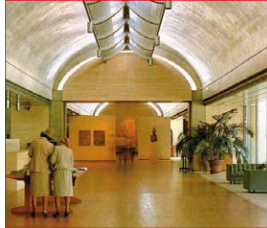
1 Regulating direct and indirect lighting in the Kimbel Art Museum in Fort Worth, Texas (arch. L.Kahn).
