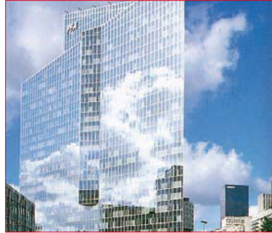
A building's solar gain can be affected if a neighbour builds one of these...
