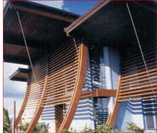
Office and workshop buildings in Baie Mahault (Guadeloupe) (arch. P. Huguet)
