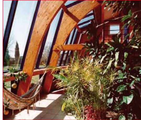
A building reacts to the climate to ensure greater comfort for its occupants (arch. Y. Célaire). 1
