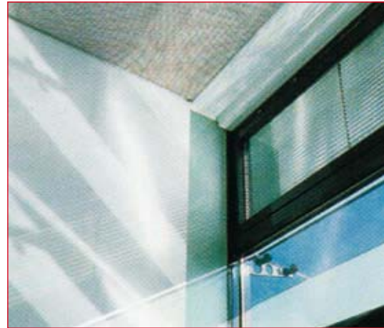
Light redirection system (Okasolar). 1
