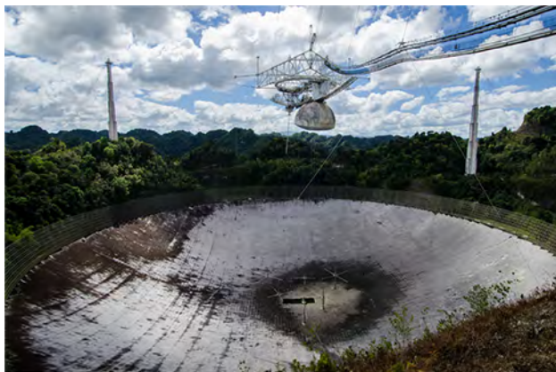
Figure 4.20 A 305-m-diameter paraboloid at Arecibo in Puerto Rico is lined with reflective material, making it into a radio telescope. It is the largest curved focusing dish in the world. Although D for Arecibo is much larger than for the Hubble Telescope, it detects radiation of a much longer wavelength and its diffraction limit is significantly poorer than Hubble's. The Arecibo telescope is still very useful, because important information is carried by radio waves that is not carried by visible light. (credit: Jeff Hitchcock)
