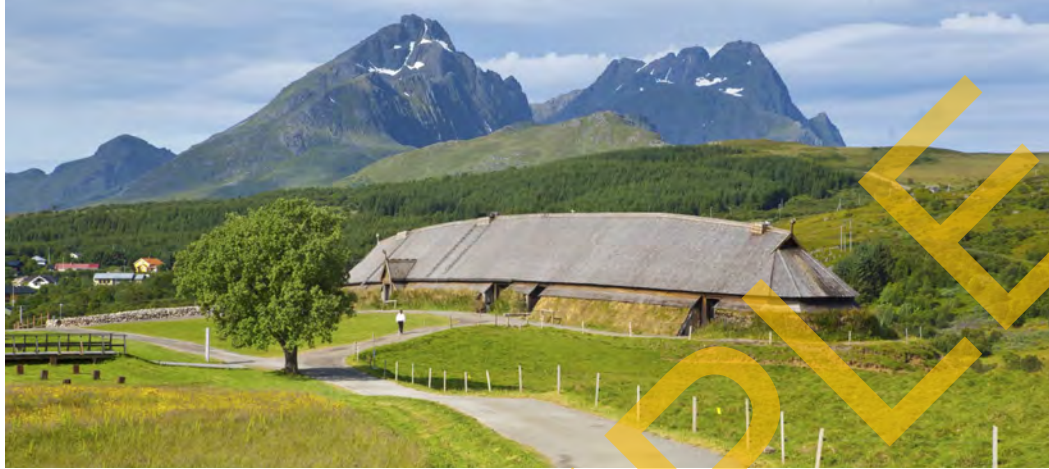
Source 7.23 A reconstruction of the 83 metre longhouse found near Lofoten, Norway. It shows how earth was piled along walls, and sometimes over the roof, to insulate longhouses.
