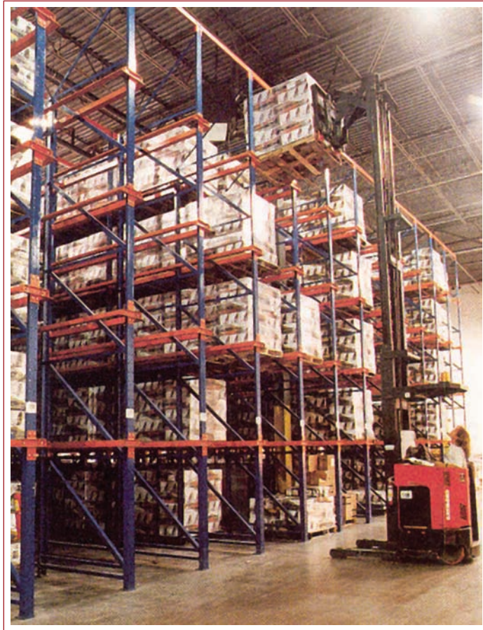
Figure 27 Seismic design criteria for steel storage racks of the type used in large warehouses and big-box retail stores are included in the Provisions .
