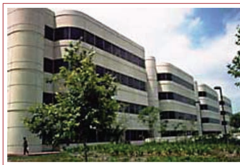
Figure 28 The San Bernardino County Justice Center in California was one of the first base-isolated buildings in the United States.
