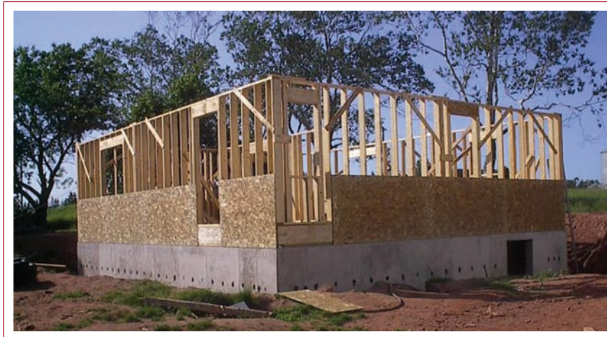
Figure 21 Wood studs and structural panel sheathing of typical wood frame bearing wall construction.
