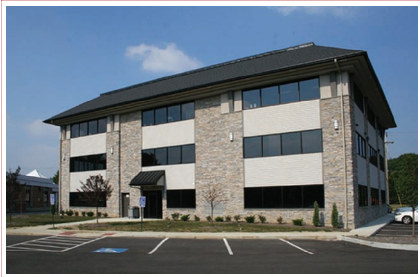
Figure 23 A three-story masonry bearing wall building.
