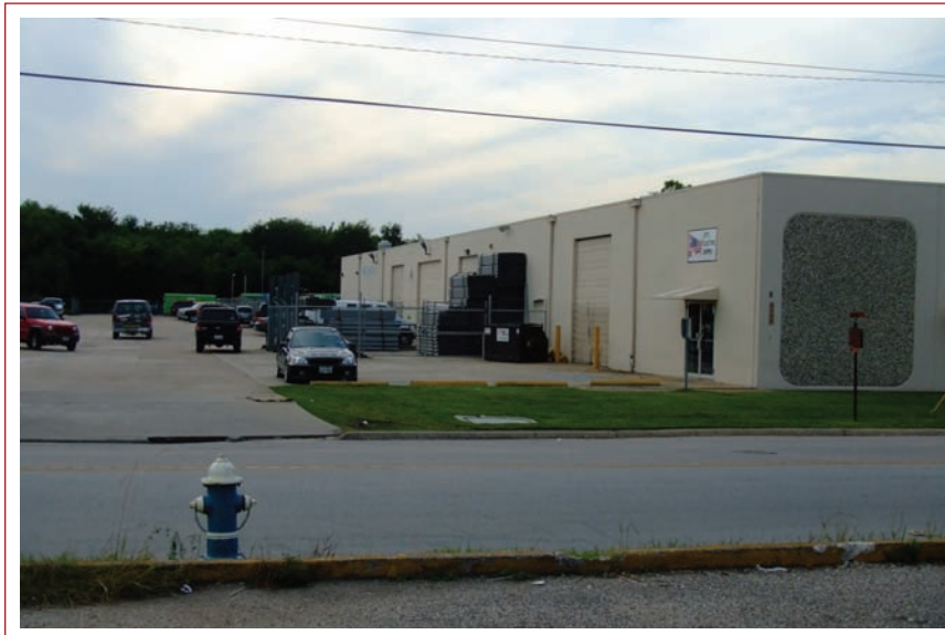
Figure 22 Typical low-rise concrete bearing wall building.
