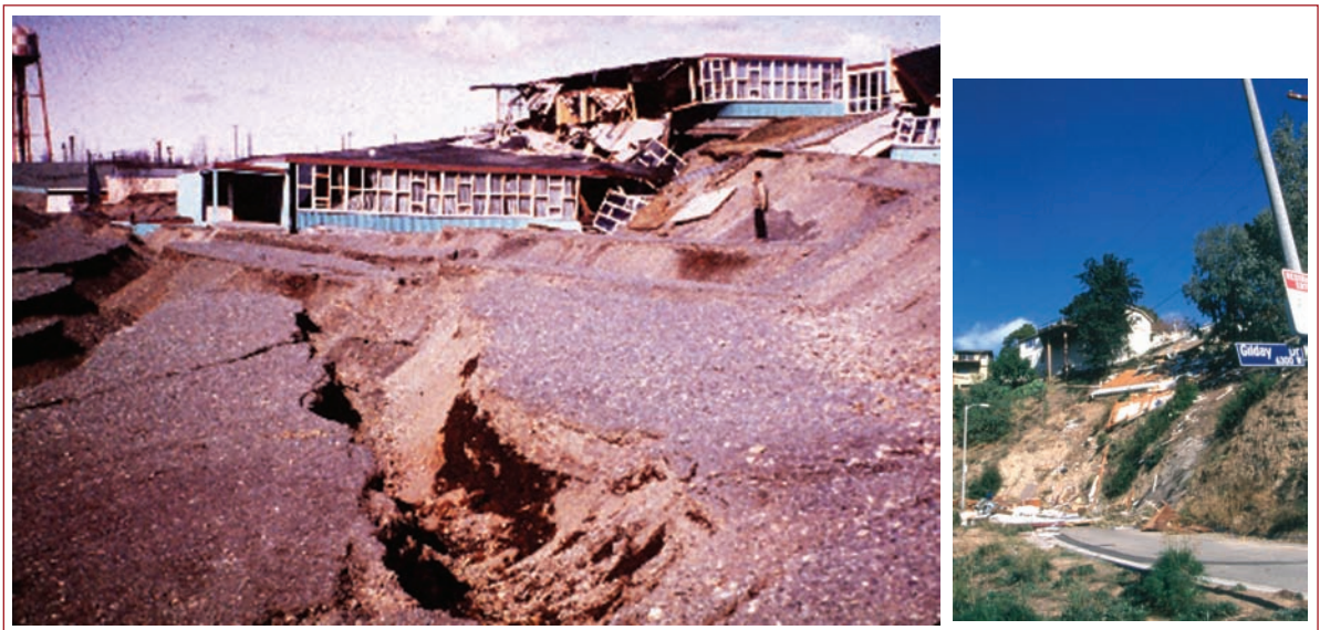
Figure 5 Earthquakes can trigger landslides that damage roads, buildings, pipelines, and other infrastructure. Steeply sloping areas underlain by loose or soft rock are most susceptible to earthquake-induced landslides. The photo on the left shows Government Hill School in Anchorage, Alaska, destroyed as a result of a landslide induced by the 1964 earthquake; the south wing of the building collapsed into a graben at the head of the landslide (photo courtesy of USGS). The home shown on the right was destroyed when the hillside beneath it gave way following the 1994 magnitude 6.7 Northridge earthquake (FEMA photo).
