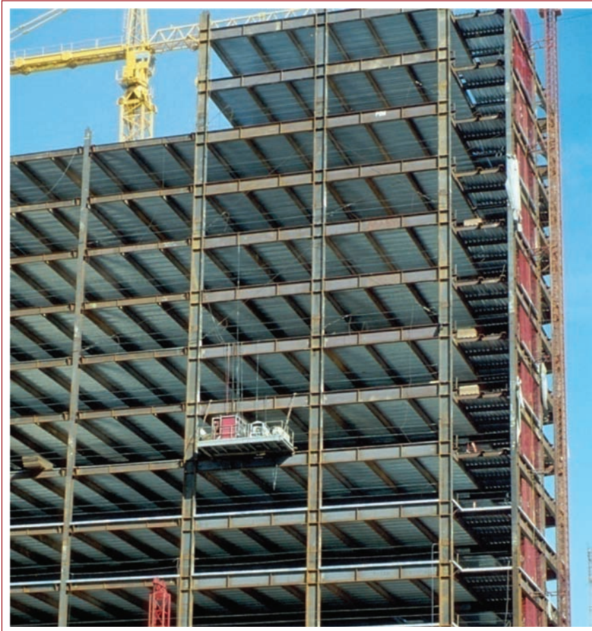
Figure 25 A tall steel moment-frame structure under construction.
