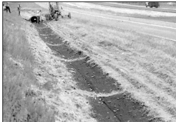
Figure 5.5. Installed TRM channel lining.
