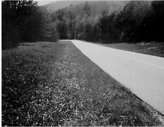
Figure 5.2. Vegetative channel lining.
