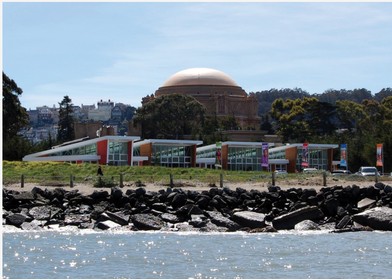
Figure 7.4 Crissy Field Center, San Francisco
