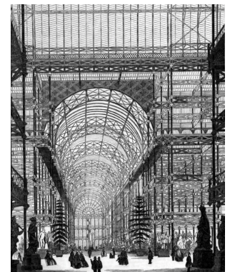
Figure 5.23 Interior of London’s Crystal Palace, the Construction of Which Was Inspired by the Leaf Structure of the Amazon Water Lily
