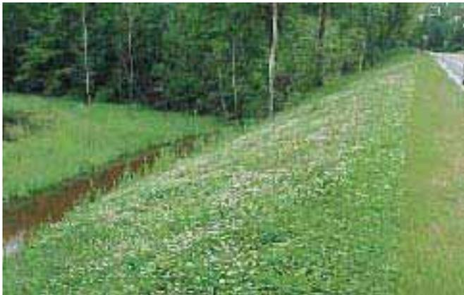
Final stabilization is achieved when all soil disturbing activity is completed and the exposed soils have been stabilized with a vegetative cover with a density of 70% over the entire site.
