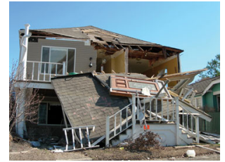
Figure 6.2 Hurricane Katrina Aftermath
