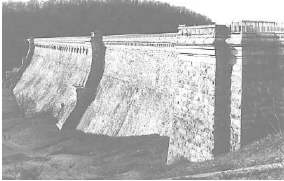
Masonry Gravity Dam (non-over flow)
