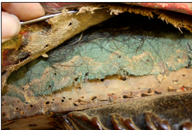
Fig. 41: Revealing horsehair padding.
