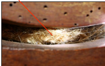
Fig. 105: Revealing tow between rails.
