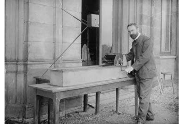
Prandtl's water tunnel, 1902.
