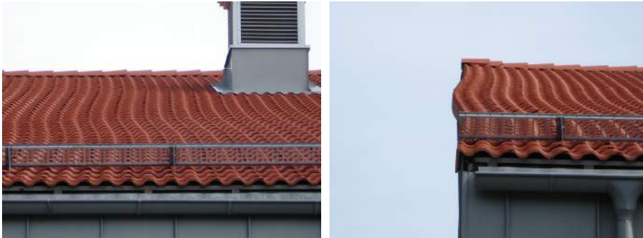
Figure 114-3. Example of deformations at failure.
