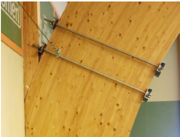
Figure 115-3. Temporary steel fixings attached to the column.
