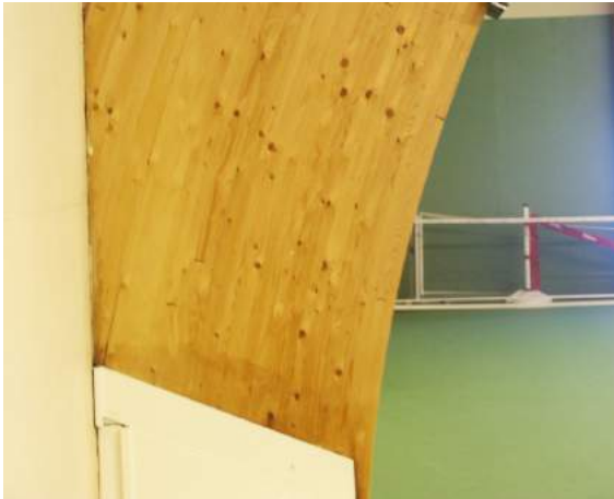
Figure 115-1. Arched column with steel parts (in white).
