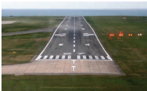
Figure 9.13: PAPI: The greater number of red lights visible compared with the number of white lights visible in the picture means that the aircraft is flying below the glide slope. Wikimedia Commons / Public domain.
