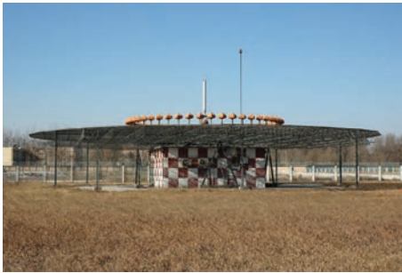
(a) D-VOR/DME ground station. © User:Yaoleilei / Wikimedia Commons / CC-BY-SA-2.0.
