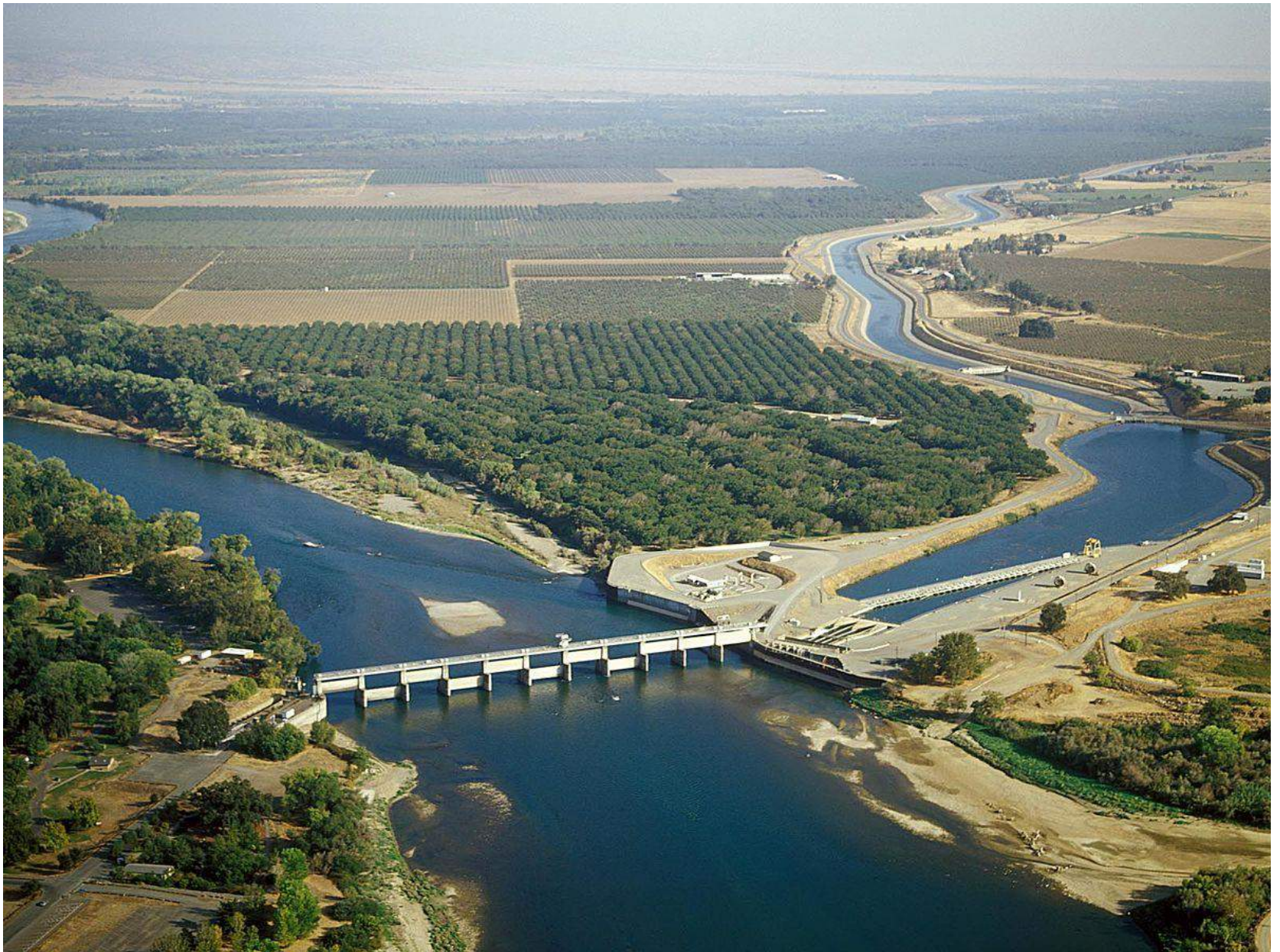
Red Bluff Diversion Dam
