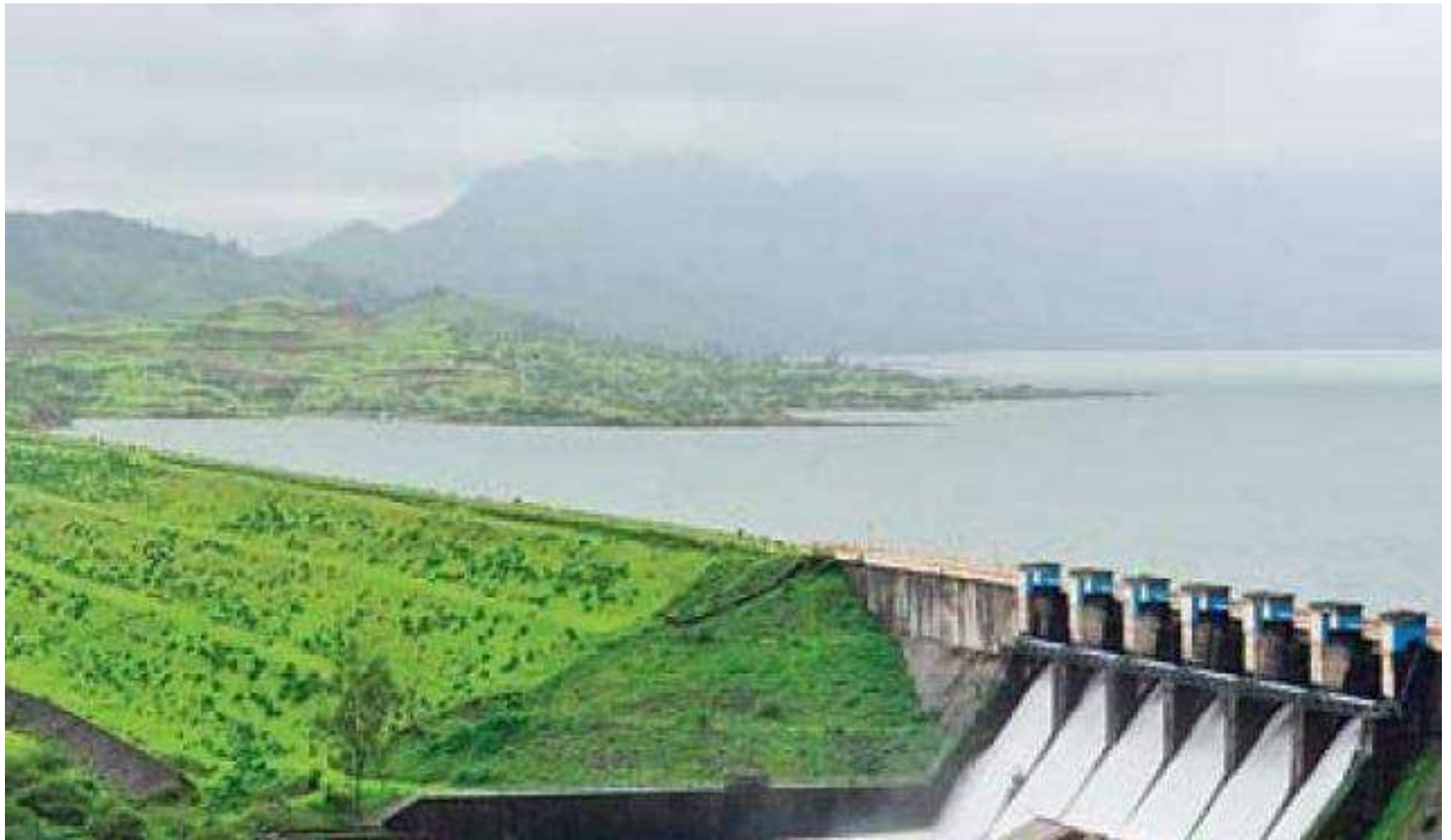
Koyna Dam, Maharashtra
