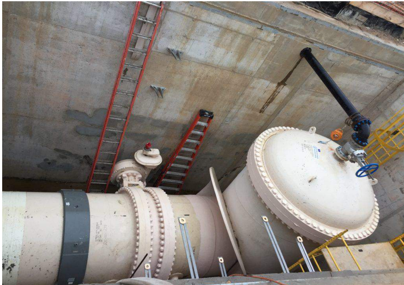
Brooklyn-to-Staten Island Drinking Water Tunnel
