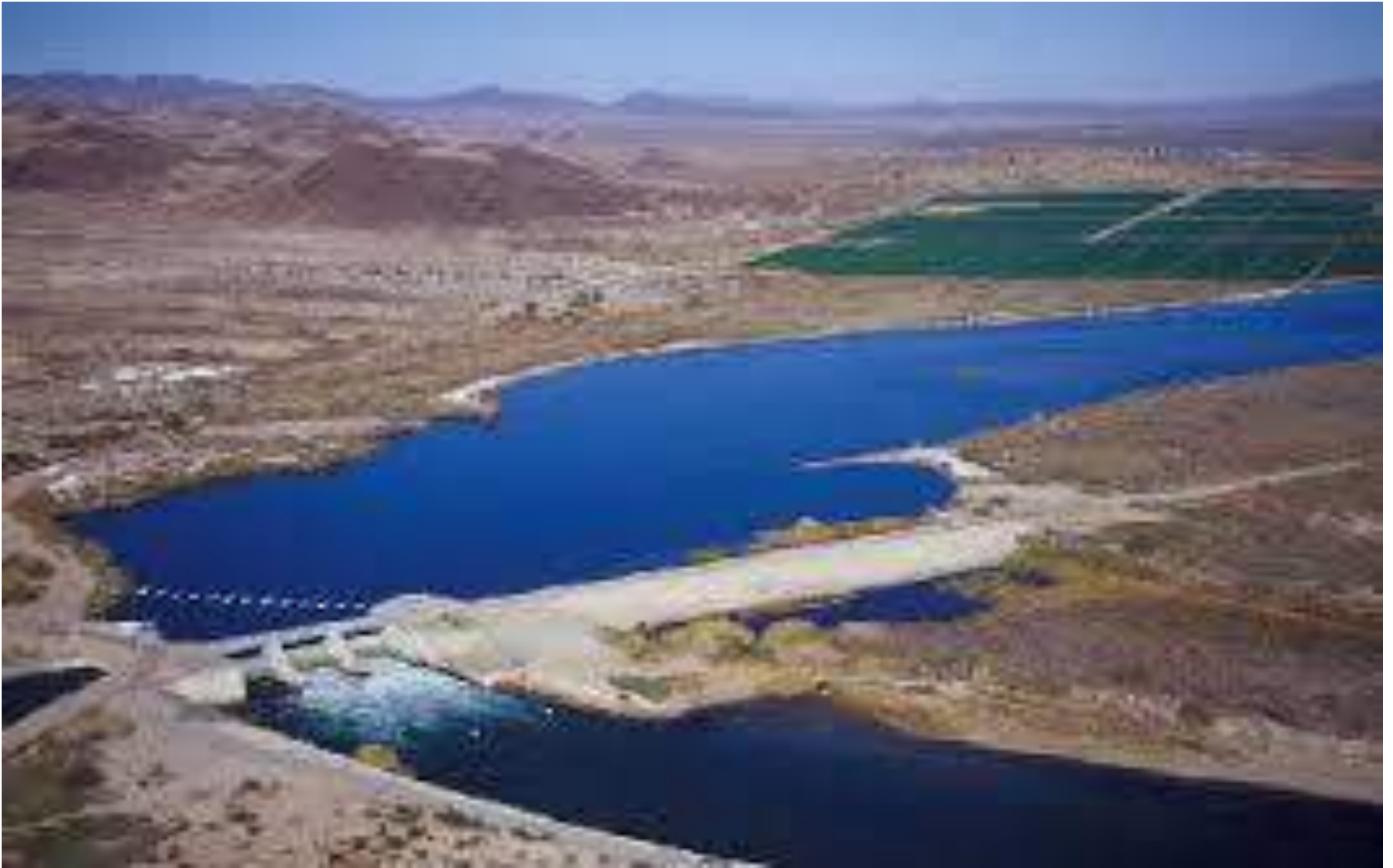
Palo Verde Diversion Dam
