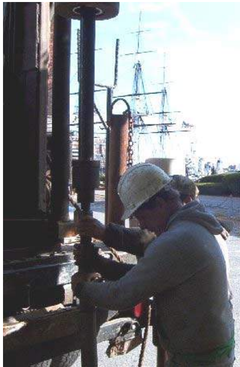
Photograph 2.2 – Standard Penetration Test
