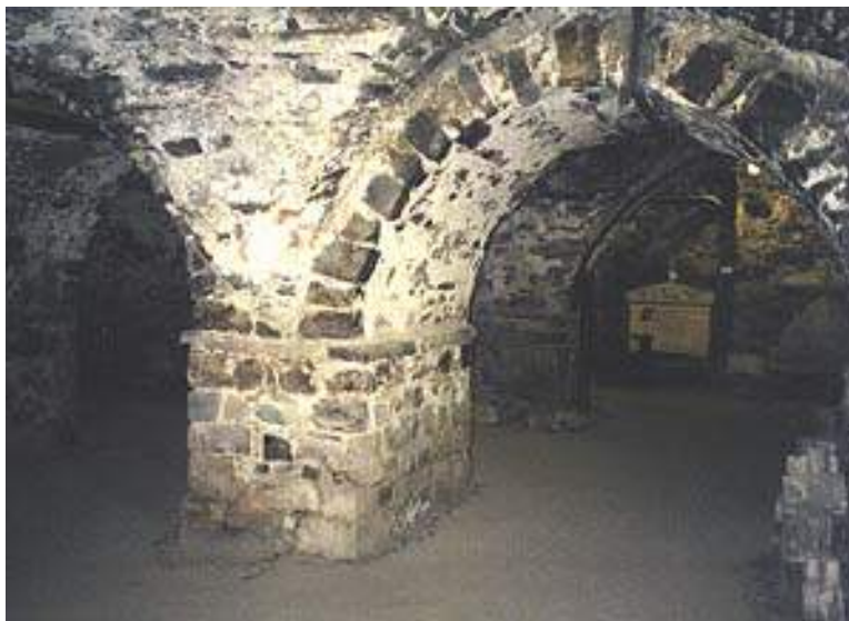
Photograph 1.1 - Foundations for a Medieval Era Cathedral
