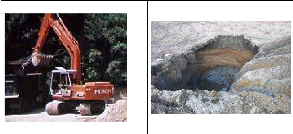
Photograph 2.1 – Test Pit Excavation
