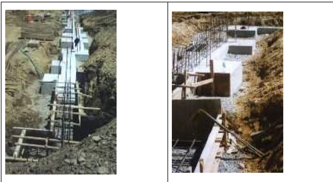
Photograph 4.1 – Shallow Spread Footings
