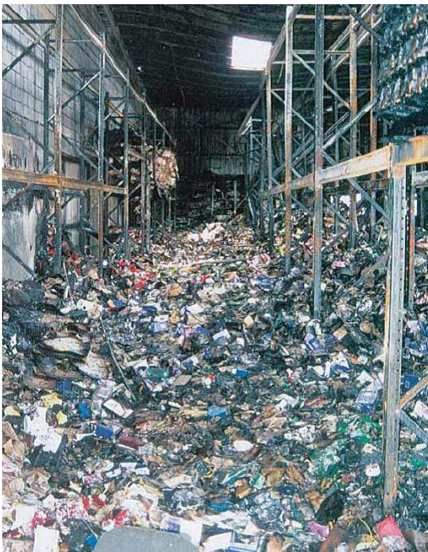
Results of a fire in a perfume warehouse (Source: Munich Re)
