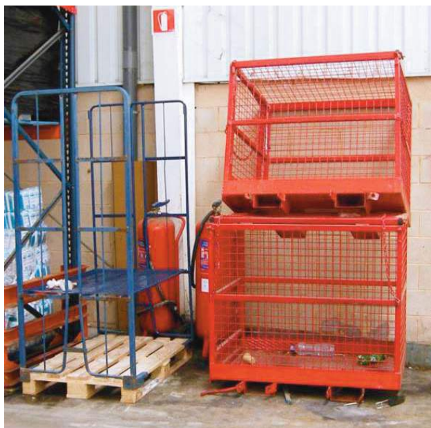
Extinguishers obstructed by loading equipment
