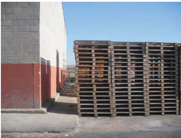
Pallet storage segregated by an exterior wall
