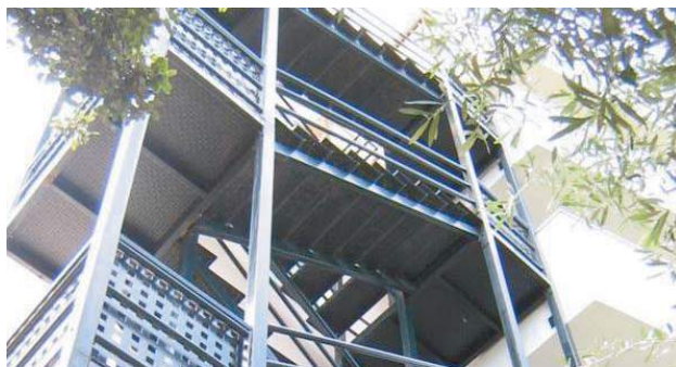
External emergency staircase
