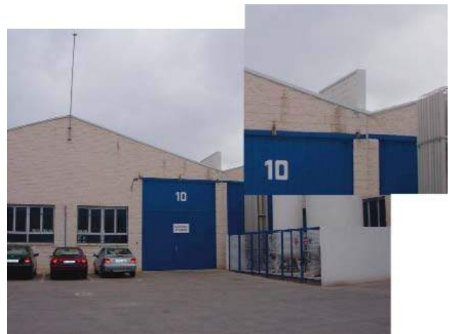
A dividing wall separating two buildings
