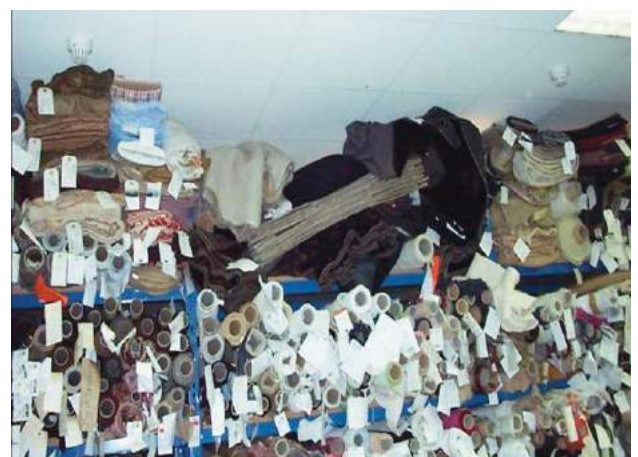
Obstructed automatic detectors
