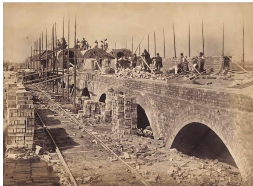
Source 5.56 The building of a London sewer, c. 1860
