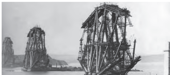
Source 5.25 The Forth Railway Bridge in east Scotland under construction. By the time of its completion in 1890, it was the longest bridge of its kind.
