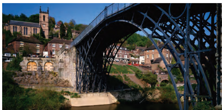
Source 5.24 This bridge in the town of Ironbridge, England, designed by Thomas Pritchard and built by Abraham Darby in 1779, is the world's first iron structure.
