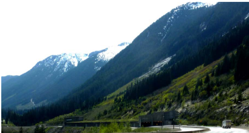
Figure 15.21 A snow avalanche shelter on the Coquihalla Highway. The expected path of the avalanche is the steep untreed slope above. [SE]
