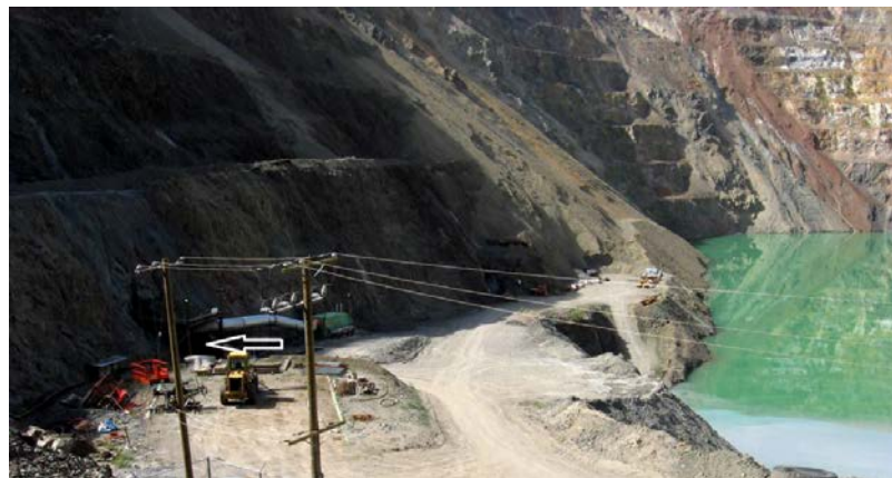
Figure 20.11 Entrance to an exploratory decline (white arrow) for the New Afton Mine situated in the side of the open pit of the old Afton Mine, near Kamloops, B.C. [SE]
