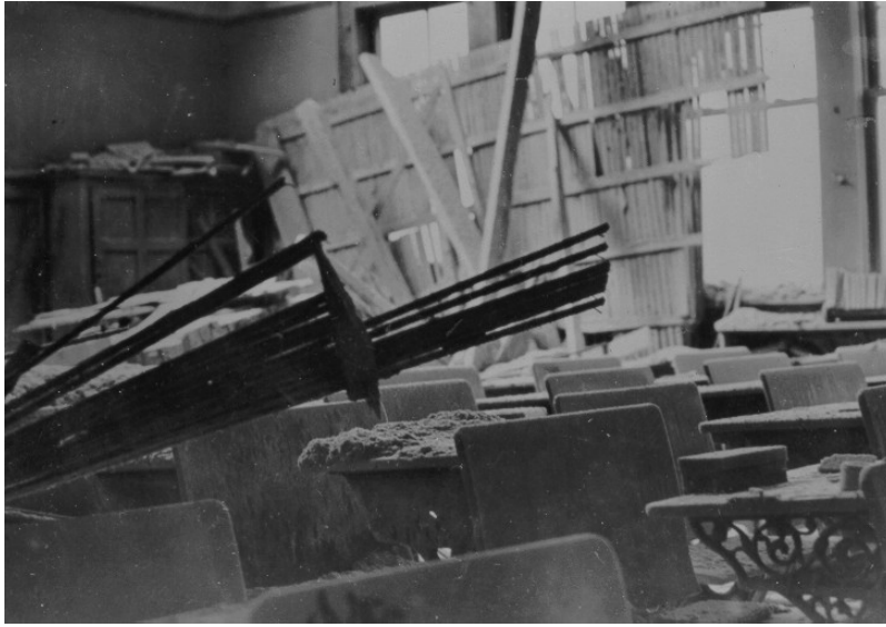
Figure 11.1 A schoolroom in Courtenay damaged by the 1946 Vancouver Island earthquake. If the earthquake had not happened on a Sunday, the casualties would have been much greater. [from Earthquakes Canada, http://www.earthquakes.canada.nrcan.gc.ca/historic-historique/events/images/19460623_1946_school.inside.jpg ]
