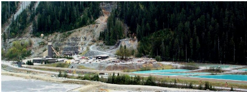
Figure 20.13 The tailings pond (lower left) at Myra Falls Mine with settling ponds (right) for processing water from the concentrator. [SE]
