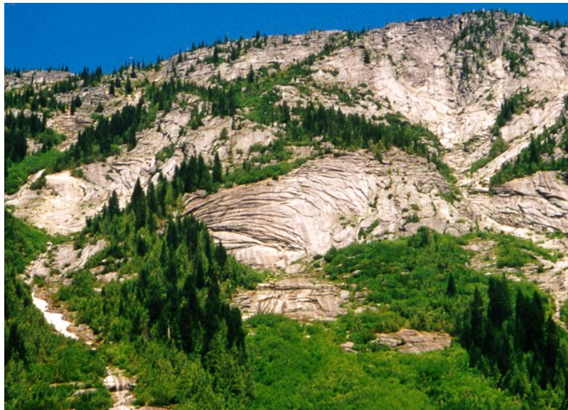
Figure 5.3 Exfoliation fractures in granitic rock exposed on the west side of the Coquihalla Highway north of Hope, B.C. [SE]
