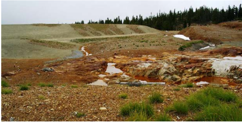
Figure 14.22 Acidic runoff at the abandoned Mt. Washington Mine near Courtenay, B.C. [SE]
