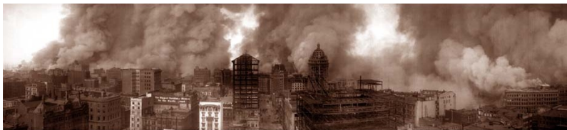
Figure 11.20 Fires in San Francisco following the 1906 earthquake. [from: http://upload.wikimedia.org/wikipedia/commons/3/3e/San_francisco_fire_1906.jpg ]
