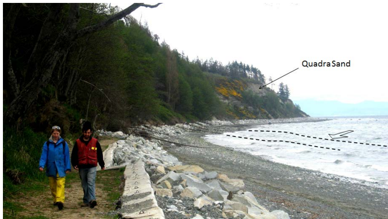
Figure 17.19 The Quadra Sand cliff at Comox, and the extensive concrete and rip-rap barrier that has been constructed to reduce erosion. Note that the waves (dashed lines) are approaching the shore at an angle, contributing to the longshore current. [SE]
