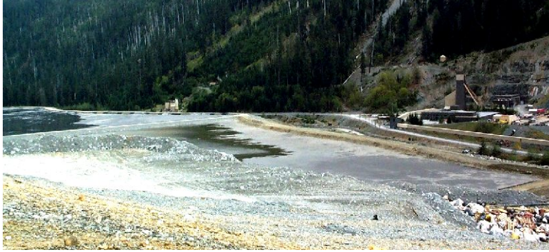
Figure 20.12 The tailings pond at the Myra Falls Mine on Vancouver Island. The dry rock in the middle of the image is waste rock. The structure on the right is the headframe for the mine shaft. Myra Creek flows between the tailings pond and the headframe. [SE]
