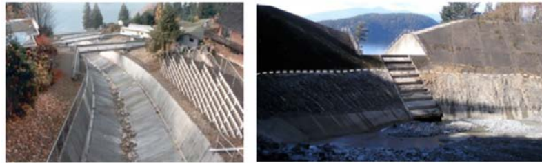
Figure 15.22 Two strategies for mitigating debris flows on the Sea-to-Sky Highway. Left: A concrete-lined channel on Alberta Creek allows debris to flow quickly through to the ocean. Right: A debris-flow catchment basin on Charles Creek. In 2010, a debris flow filled the basin to the level of the dotted white line. [SE]
