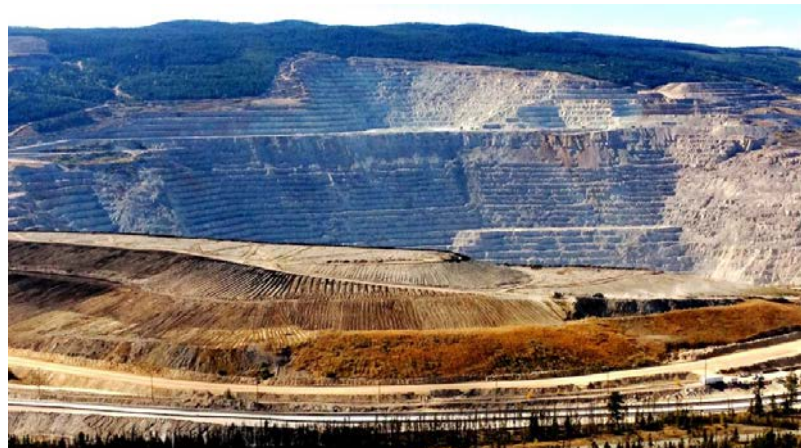
Figure 20.1 The open pit (background) and waste-rock piles (middle) of the Highland Valley Copper Mine at Logan Lake, British Columbia [Photo by Russell Hartlaub, used with permission]
