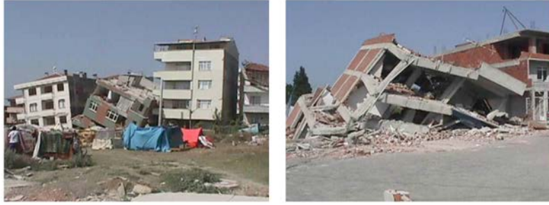
Figure 11.18 Buildings damaged by the 1999 earthquake in the Izmit area, Turkey. [from U.S. Geological Survey at: http://gallery.usgs.gov/sets/1999_Izmit_Turkey_Earthquake/thumb/_/1 ]
