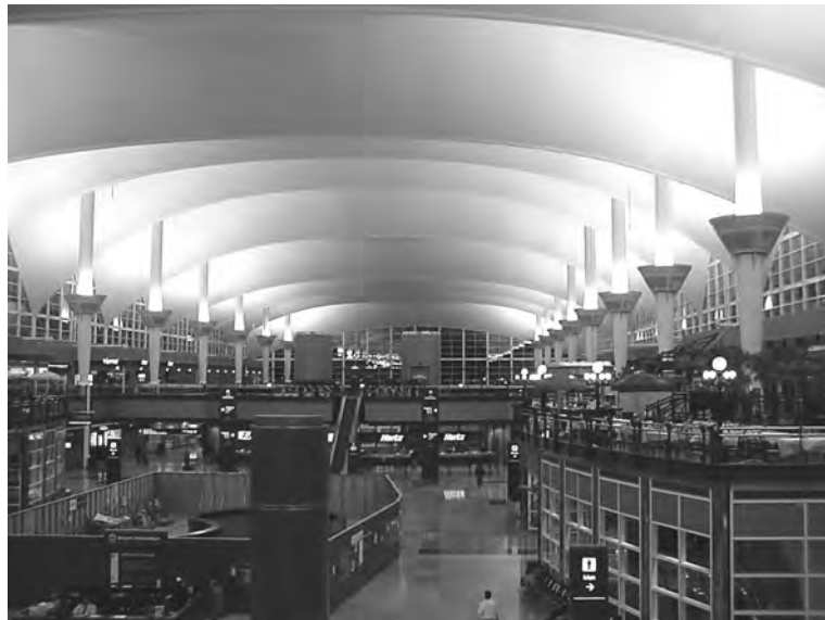
FIGURE 1-2 Tension fabric roof at the Denver International Airport.
