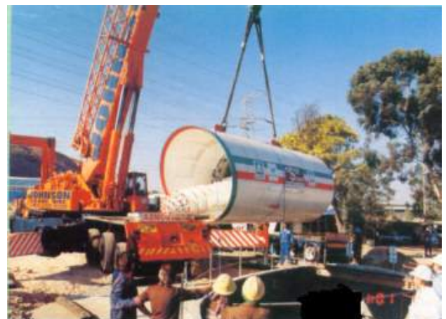
Fig. I-6. In-shield boom cutter (type of road header cutter boom mounted in a shield) (©TBM Exchange Int., 2002)
