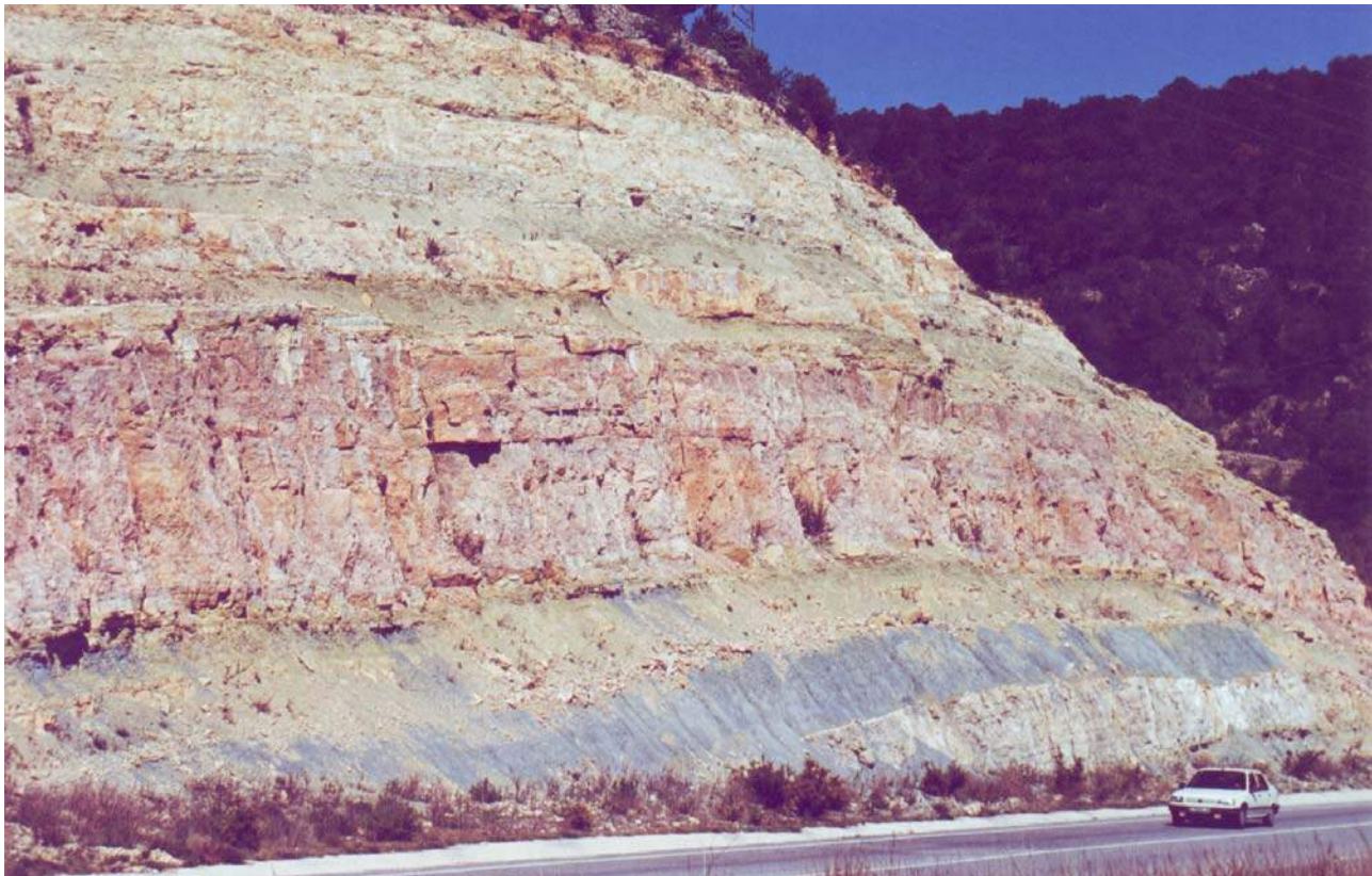
Fig. A-6. Different geotechnical units present in a single slope. Greenish and bluish gray layers consist of calcareous shale and brownish, pinkish off-white layers consist of dolomite and limestone.
