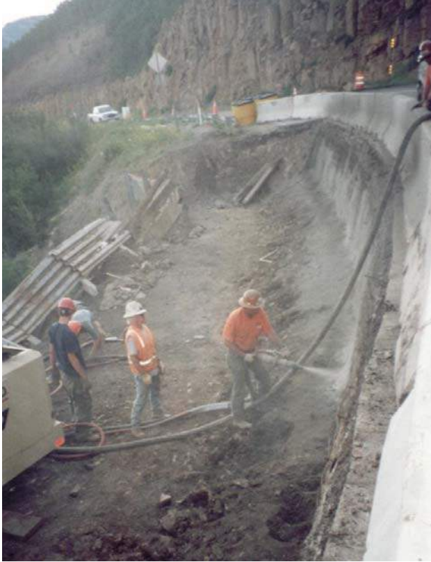
Fig. J-6. Shotcrete applied at a road site (Battle Mountain, Colorado, USA; photo courtesy: Alyssa Kohlman)
