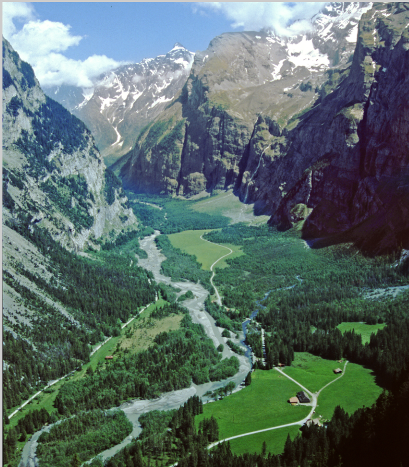
Fig. 1.4. The glaciated trough of the Gasterntal, looking up-valley from the Stock hill; the 1908 tunnel breakthrough created a valley-floor sinkhole in the woodland just beyond the furthest of the large open meadows (© Tony Waltham Geophotos Ltd).
