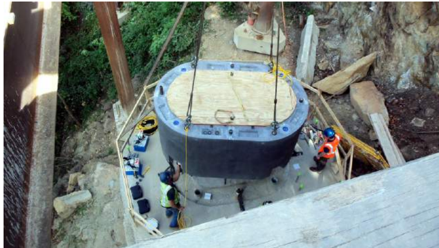
Figure 1.32 - Precast Hollow Segmental Piers, Foothills Bridge No. 2
