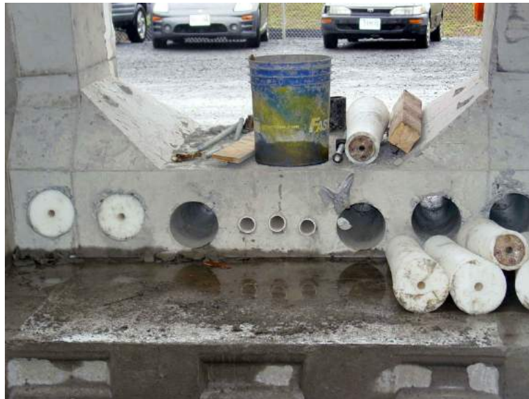
Figure 2.12 - Reusable Diabolo Inserts at Deviation Segment
