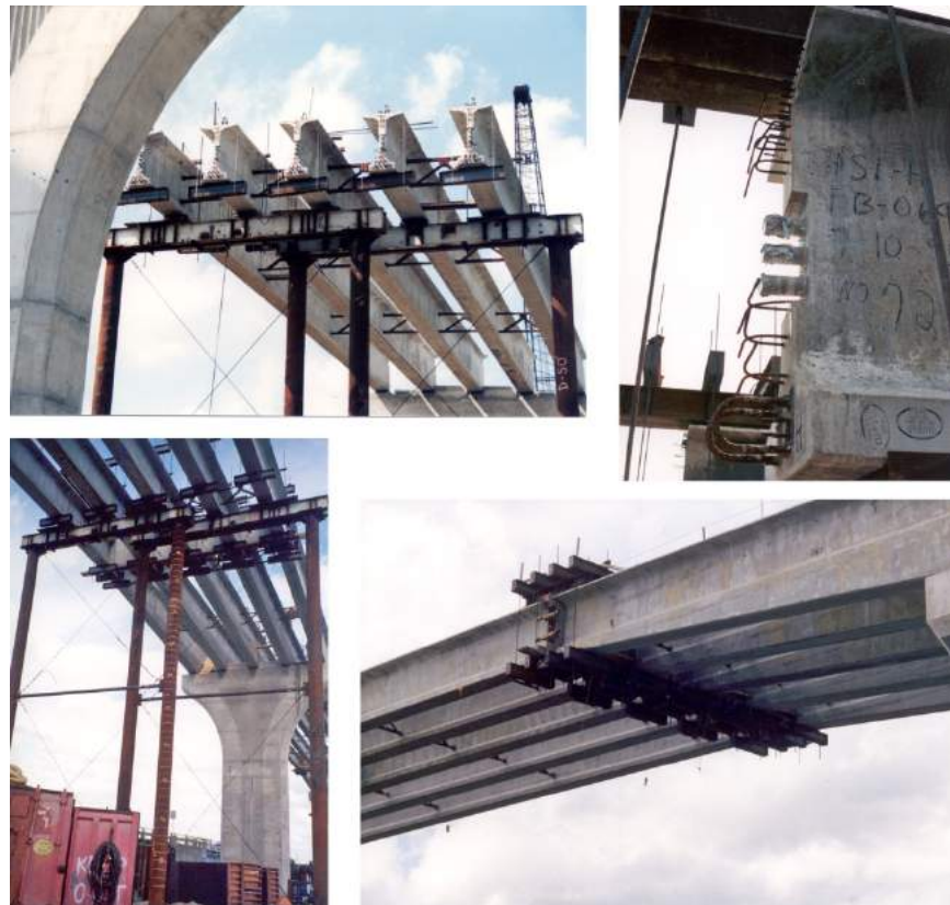
Figure 1.7 - Spliced Haunched I-Girder of Main Span Unit
