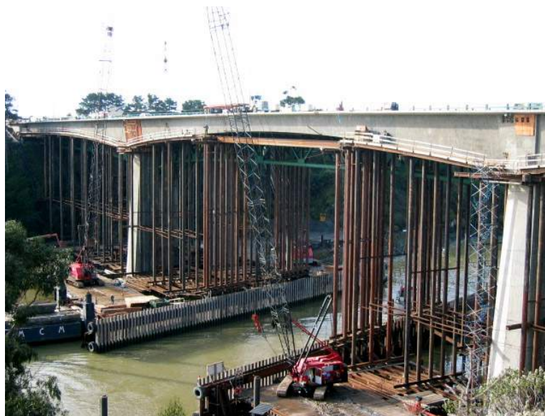
Figure 1.6 - Cast-In-Place Post-Tensioned Construction in California
