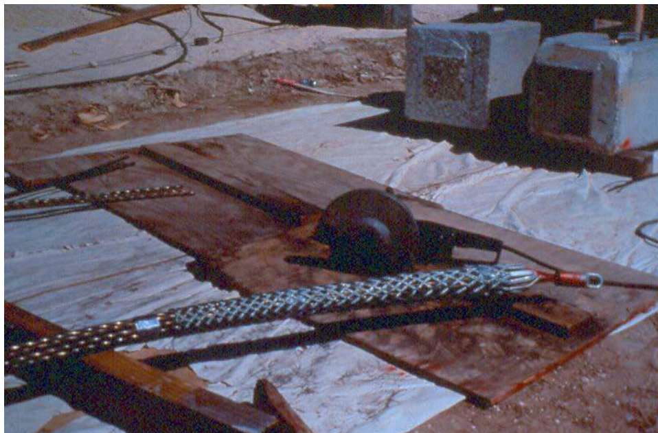
Figure 3.26 - Steel wire sock for installing multi-strand tendon
