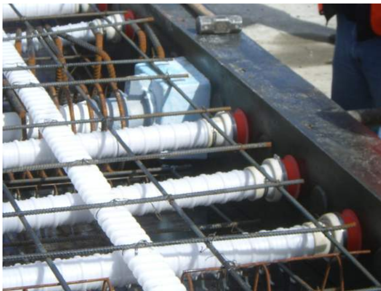
Figure 2.10 - Duct Couplers in Precast Segmental Construction
