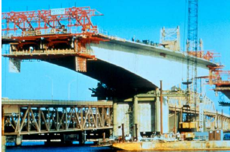
Figure 1.17 - Cast-In-Place Segmental Construction using Form Travelers
