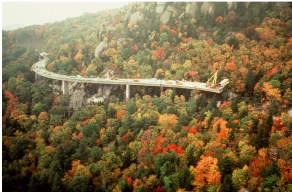
Figure 1.23 - Progressive Construction of the Linn Cove Viaduct
