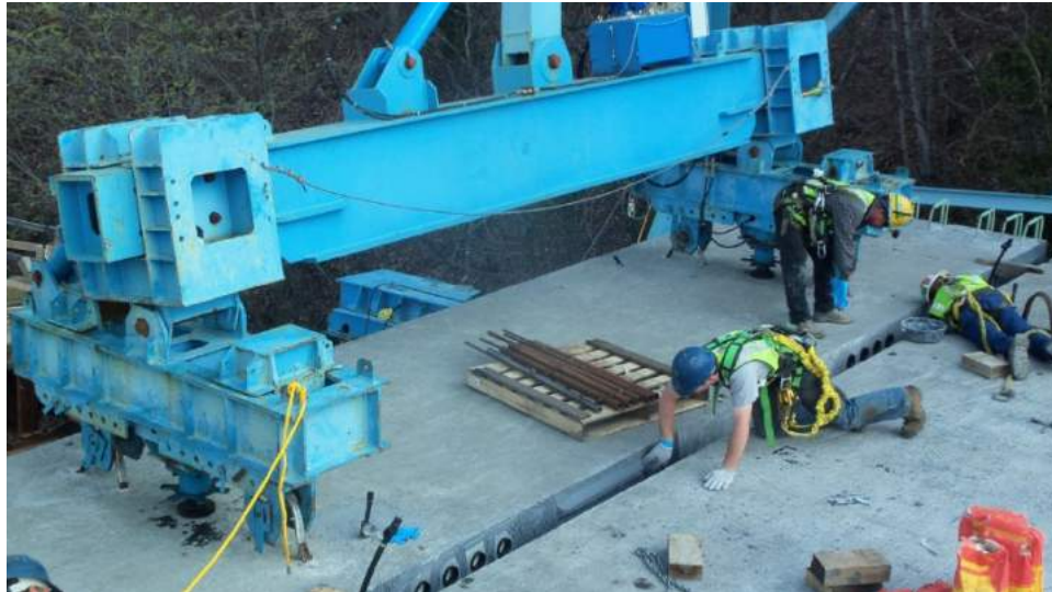
Figure 1.35 - Applying Epoxy between Precast Segments at the Foothills Parkway Bridge No. 2
