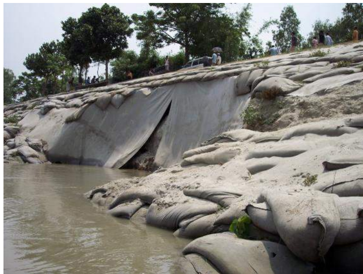
Figure 2.6: Poor performance of sand bags against cyclonic storm surge (Islam and Arifuzzaman, 2010)
