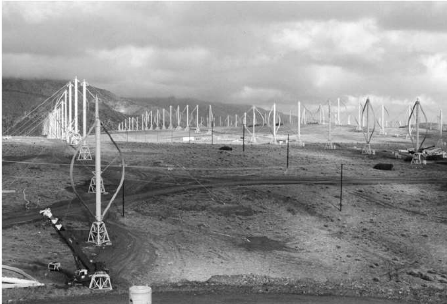
Figure 2.46. Flowind wind farm with vertical axis Darrieus turbines on the Tehachapi Mountains, 1986
