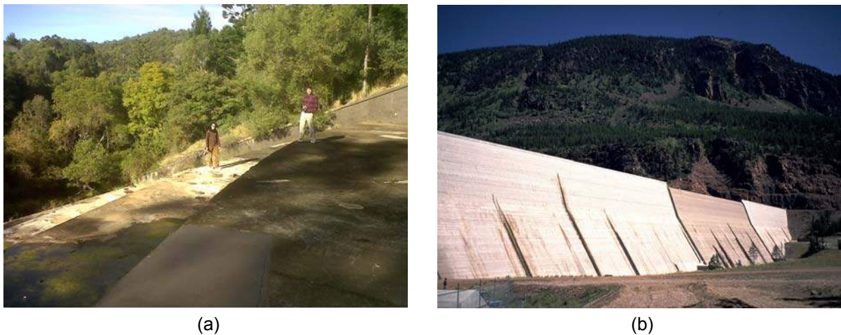
Figure 1 – Examples of emblematic stepped spillways built in the 19 th and 20 th centuries: (a) Gold Creek dam, Australia, earthen dam with a concrete stepped waterway (completed in 1885, stepped waterway built in 1890) (Photograph taken on July 2011); (b) Upper Stillwater dam, USA, RCC gravity dam with incorporated spillway, finished in 1987 (Courtesy of P. Guedes de Melo)
