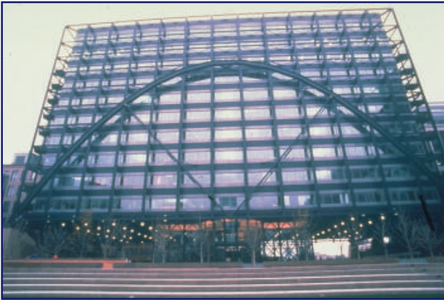
T2c161 First Exchange House (Broadgate fase 11), Londres, Reino Unido
