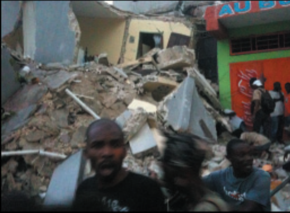
This photo provided by Carol Pedro shows people sifting past rubble of a damaged building in Port-au-Prince, Haiti, Tuesday, Jan. 12, 2010. The largest earthquake ever recorded in the area shook Haiti on Tuesday, collapsing a hospital where people screamed for help. (AP Photo/Carol Pedro)
