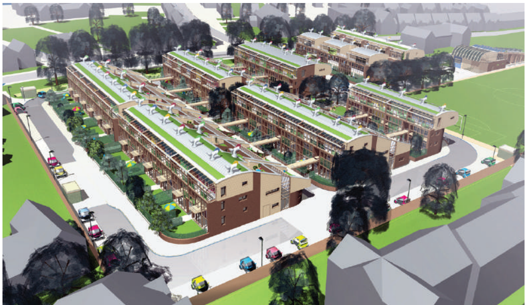
→ 'BedZed' residential scheme, London. The site layout is planned to optimise orientation for solar gain.
