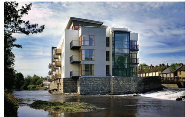
↑ This scheme makes use of a waterside location to produce a landmark with a high level of amenity for residents at Baltinglass, Co. Wicklow.
