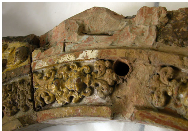
Figure 7. The key-stone arch. The classical winding acanthus leaves and vase are moulded decoration elements adhered to the modelled arch. © IMC-DGPC
