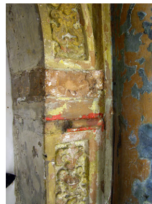
Figure 8. Incise lines are visible marking the position where the frieze moulded frieze decoration should be adhered. © IMC-DGPC
